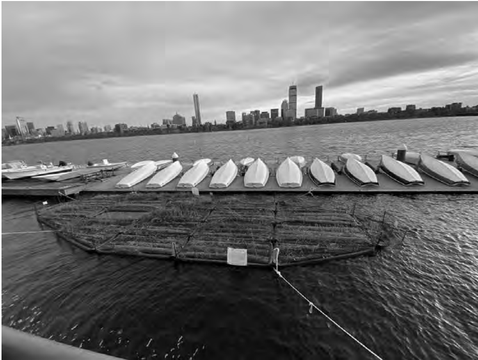
1.5 An example of resilient design: experimental floating wetlands on the Charles River, Boston, designed to suppress algal blooms. Constructed by Northeastern University. Source: Photo by Orit Halpern, December 30, 2020.
