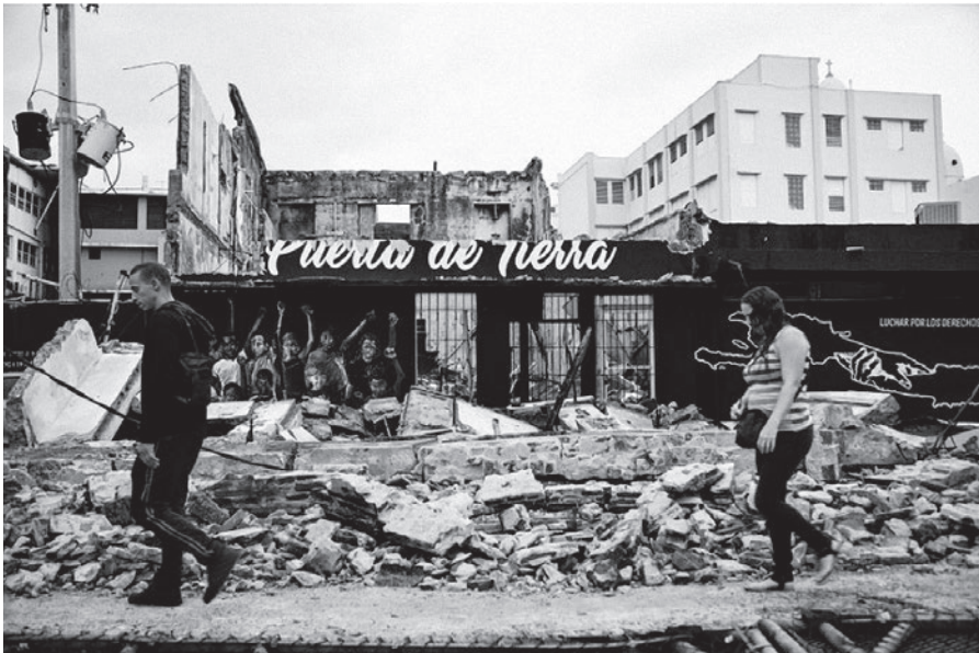
Fig 3: Puerto Rico destruction after Hurricane Maria.
